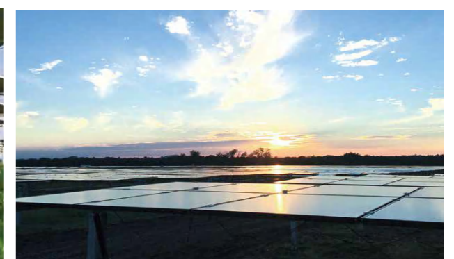
Capacity: 200MWp Location: USA Application: V-Link Tracker
