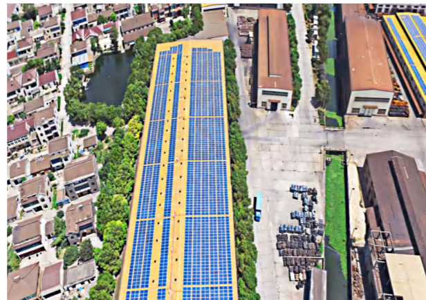
Capacity: 21.5MWp Location: Jiangsu, China Application: Metal Sheet Roof
