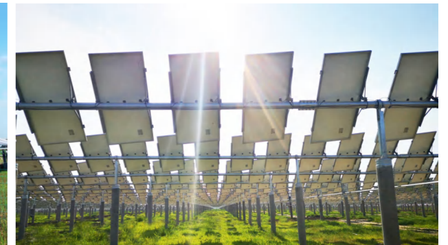
Capacity: 100MWp Location: Jilin, China Application: V-Link Tracker
