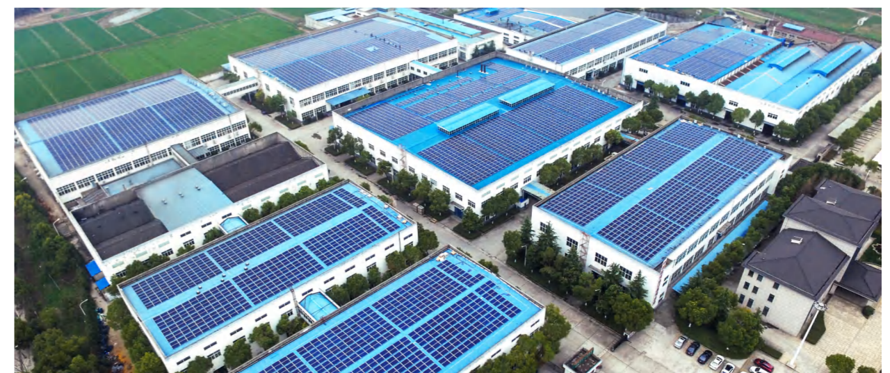
Capacity: 5.5MWp Location: JiangSu
