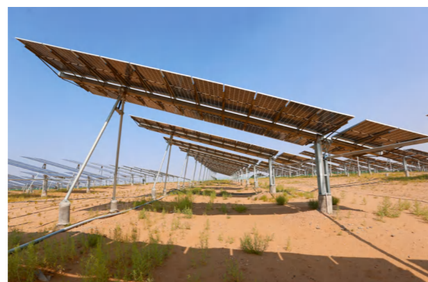
Capacity: 115MWp Location: Neimeng, China Application: Tilt Single Axis Tracker
